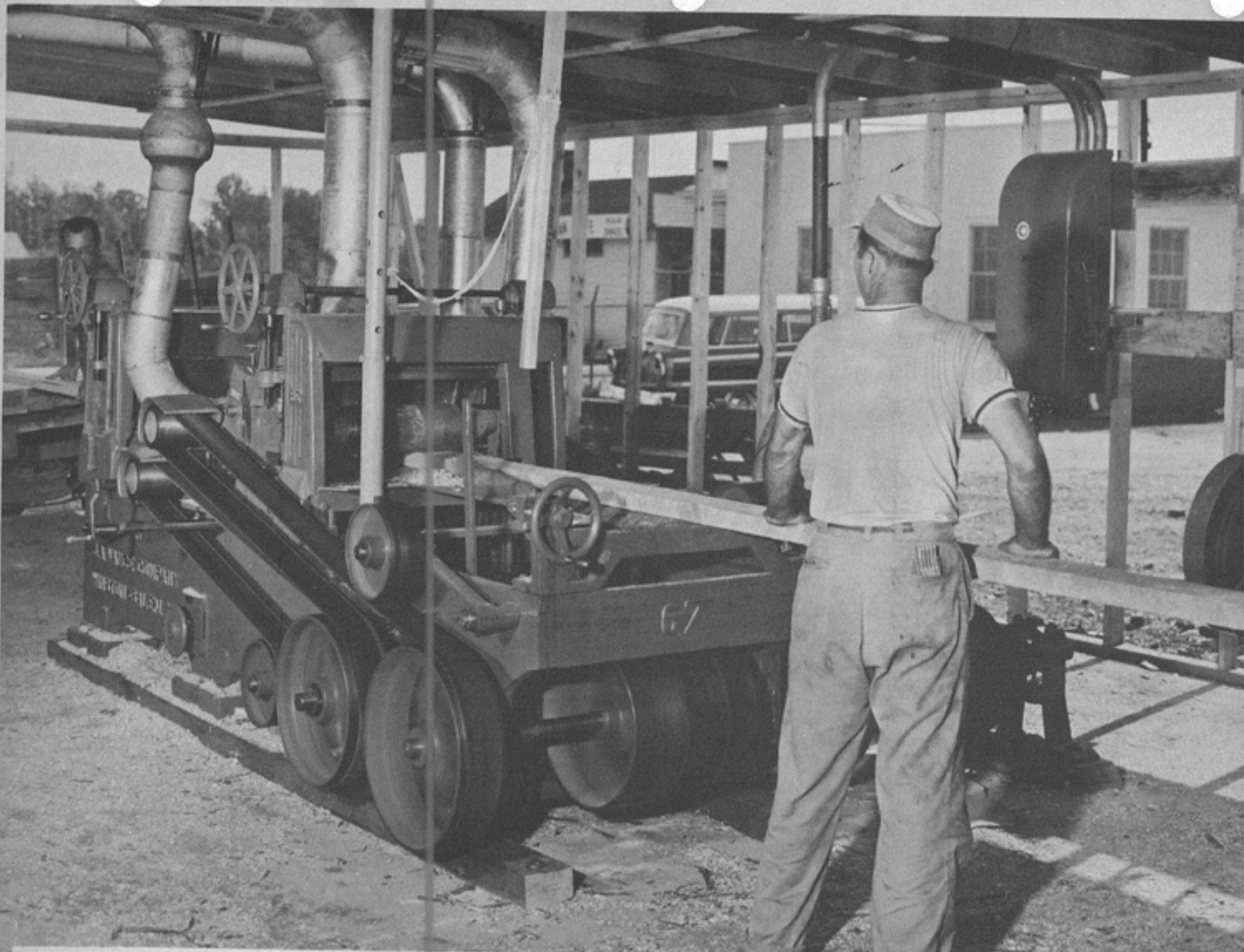
Finishing Framing on the NO. 67 VANCE DOUBLE SURFACER AND MATCHER BRUCE SMITH LBR CO. LEXINGTON, N. C.
